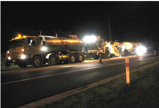
Figure 4: SH16 FBS – note cement spread on existing OGPA surfacing
