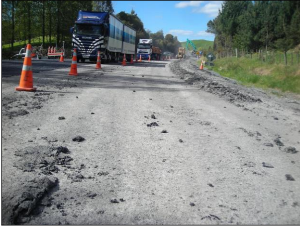
Figure 13: Removal of all seal
