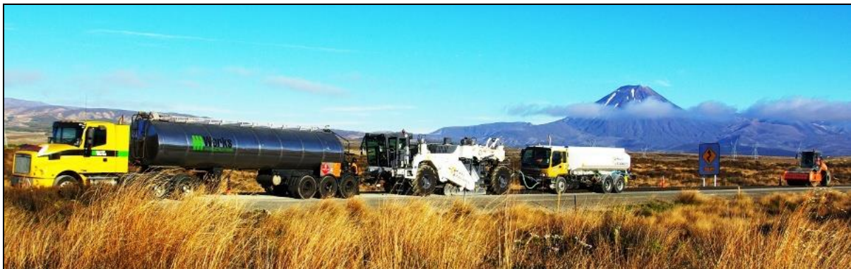
Figure 1: FBS 'train' operating in Tukino, Central Volcanic Plateau, New Zealand.
