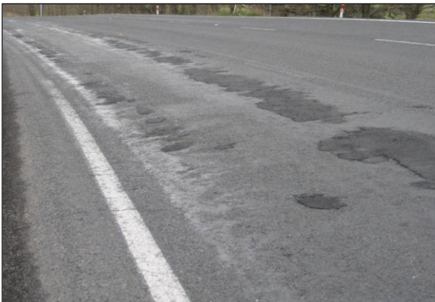
Figure 11: June '07 Primary wheel track repairs
