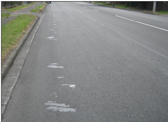
Figure 7: Membrane seal ‘bleeding’ through thin asphalt surfacing. Note line of ‘blooms’
