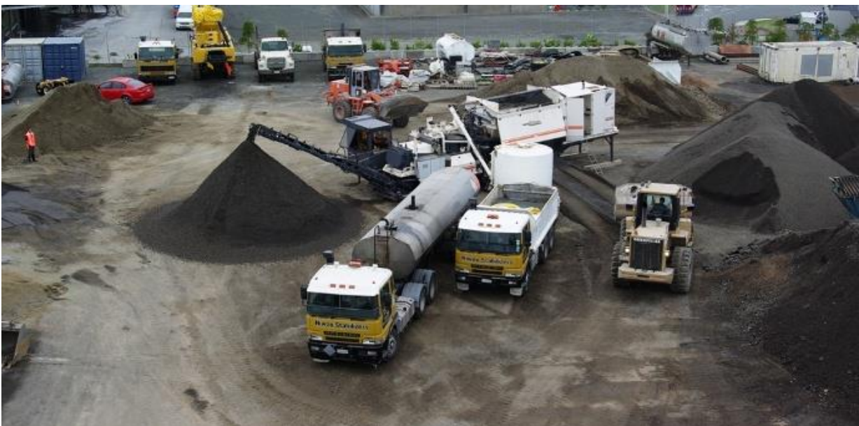
Figure 15: Ex-situ FBS basecourse production trials
