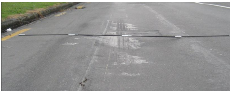
Figure 7: Membrane seal ‘bleeding’ through thin asphalt surfacing. Note line of ‘blooms’
