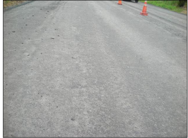
Figure 14: Exposed FBS basecourse prior to reseal
